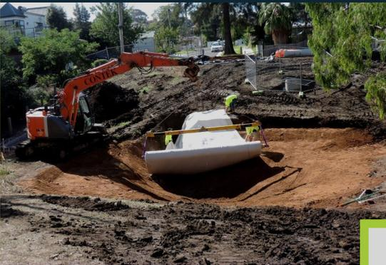
The new gross pollutant trap will remove litter from the storm water before it enters the pond. A valve can divert excessive flows back to the main drain to the creek.
