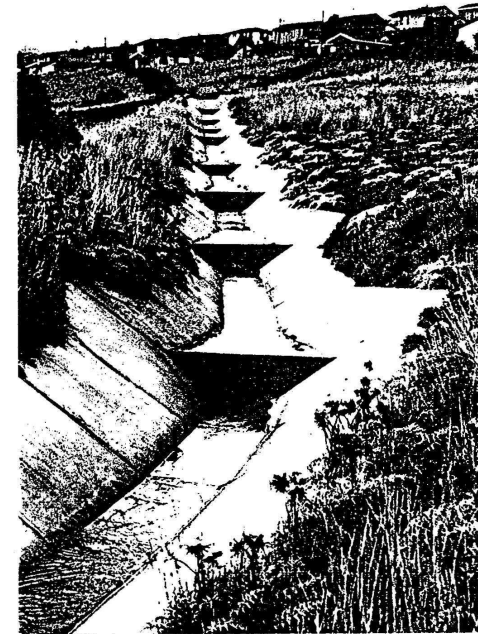
PLATE 8-13 The Railway Crescent Diversion Drain downstream of Ripplebrook Drive
