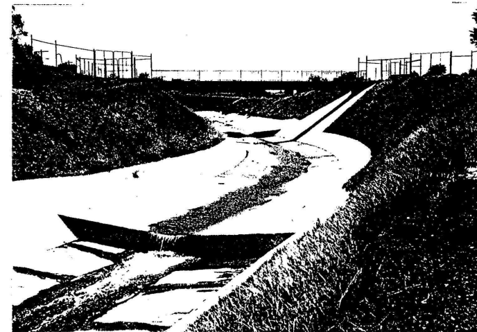
PLATE 8-6 Energy dissipating drop structures near Adelaide Street
