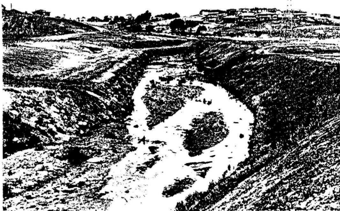
PLATE 8-12 Bank protection works downstream of Lyons Street, Broadmeadows
