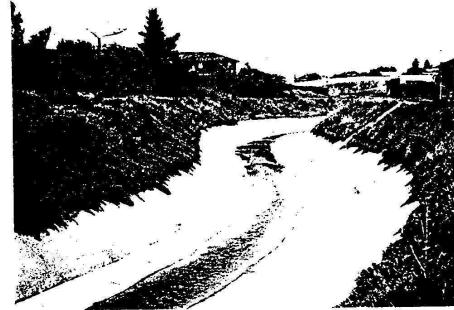
A Looking downstream from Albion Street Bridge (Type Section 1)
