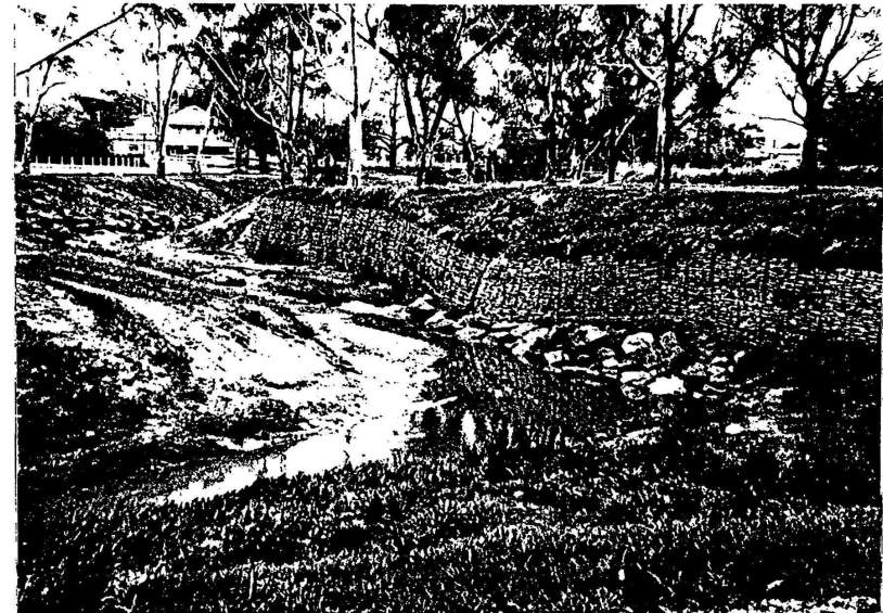
D View of the gabions in August 1980
