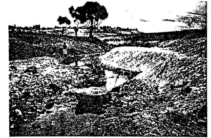
D Rocks, gravel and sand deposited along the improved channel during the Easter 1977 flood
