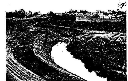
E The same view in mid 1980. Note the rock lining
