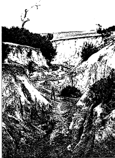
A The deeply incised middle section of the watercourse
