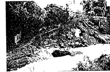
B Eroded bank and collapsed gabion, May 1974
