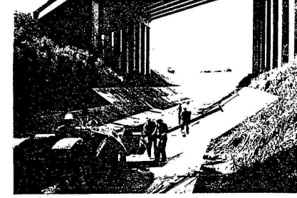
D Raising the concrete lining under the Tullamarine Freeway at Bell Street
