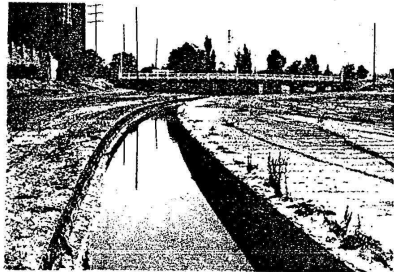
C The berms downstream of Racecourse Road immediately after regrading
