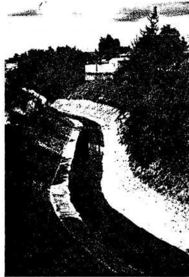
PLATE 5-12 Improvements at Donald Avenue: View looking downstream from Morrow Street in March 1980
