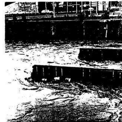
PLATE 5-20 The timber training walls on the upstream side of Flemington Road Bridge
