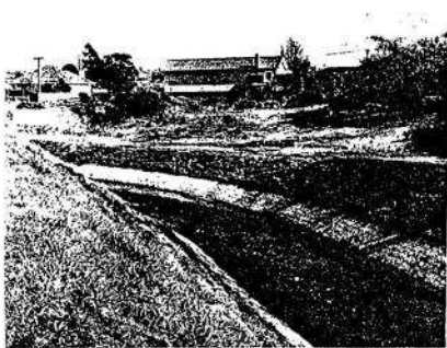
C View looking downstream in 1960 immediately after completion of improvement works
