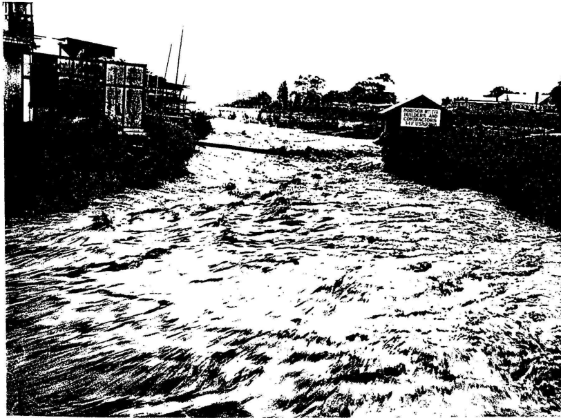
A Floodwaters racing through the constricted channel above Flemington Road Bridge
