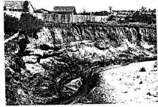
A Bank erosion, 1955
