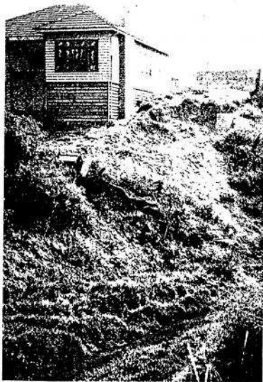
PLATE 5-10 House sited near the bank edge, Morrow Street, Brunswick
