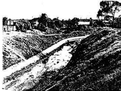
D View looking upstream in 1960 immediately after completion of improvement works
