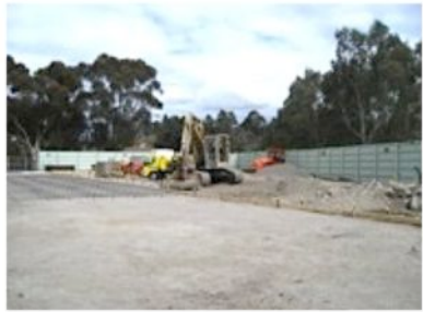
Northern Sewerage Project site, when work started in 2008
