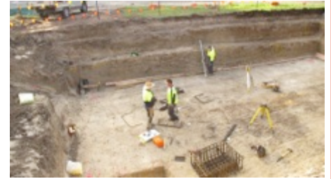
The serious tank being constructed under Napier Park
