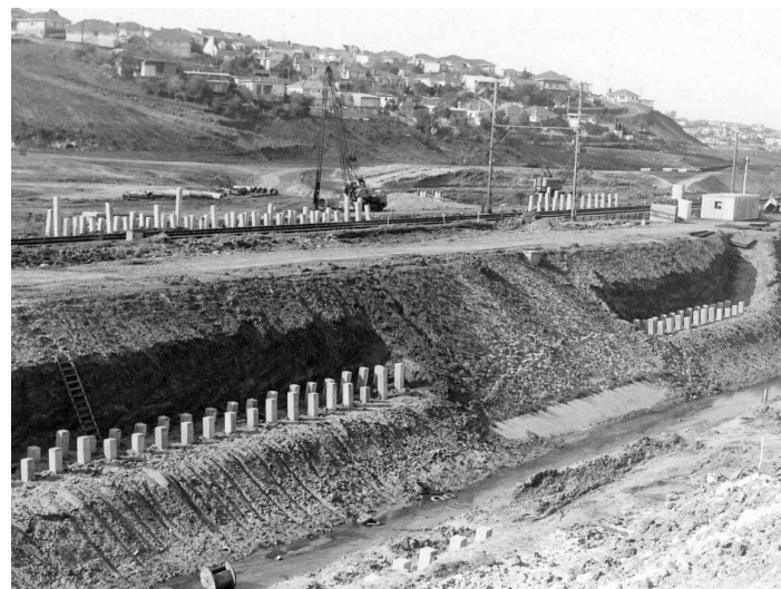
Pylons for Bell St interchange, 1968. Ruby Brideson
