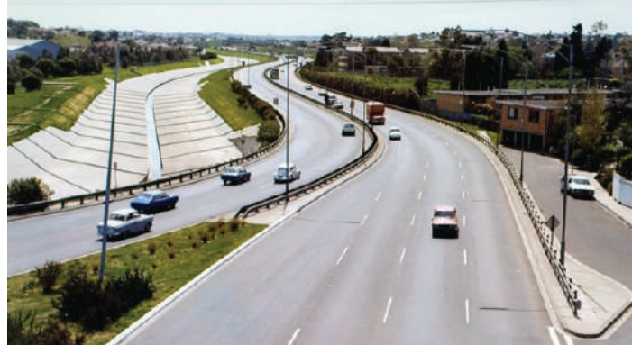
Wide Channel pre-concrete, and the final result, 1970
