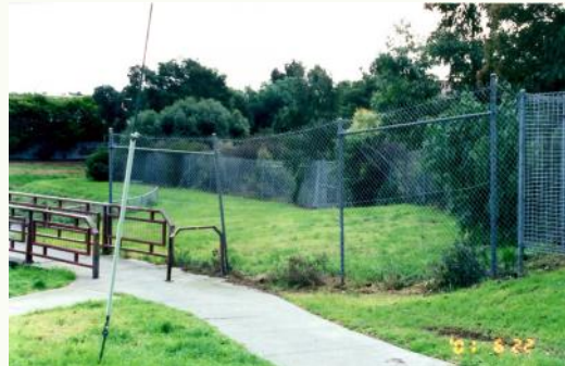
Gaffney St Bridge
