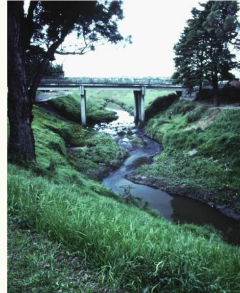
Moreland Road Bridge
