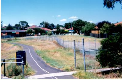
Talbot Road Bridge
