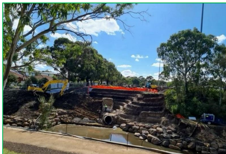
Construction of pond and terracing in progress.
