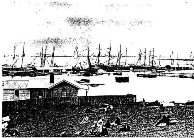
D View from Batmans Hill looking south-westwards towards Williamstown. The ships mark the line of the Yarra River
