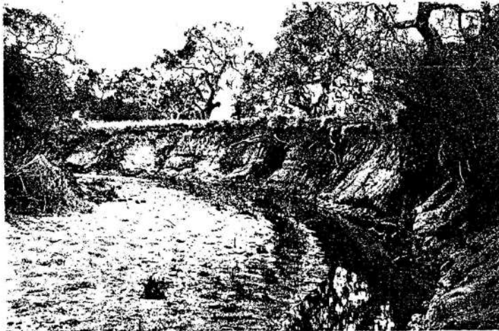
PLATE 1-1 Erosion along Moonee Ponds Creek near Oaklands Junction
