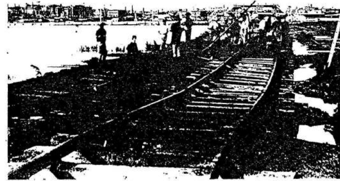
C The damaged Melbourne-Sandridge railway line
