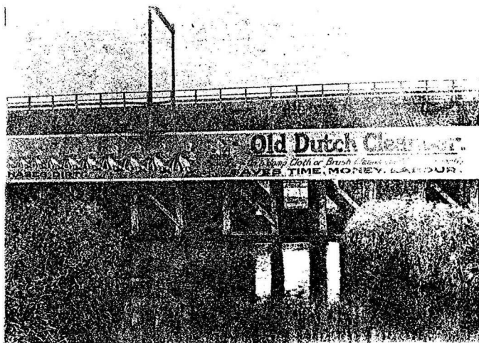
A—View looking downstream towards the bridge. Note the dense growth of vegetation along the sides of the channel.
