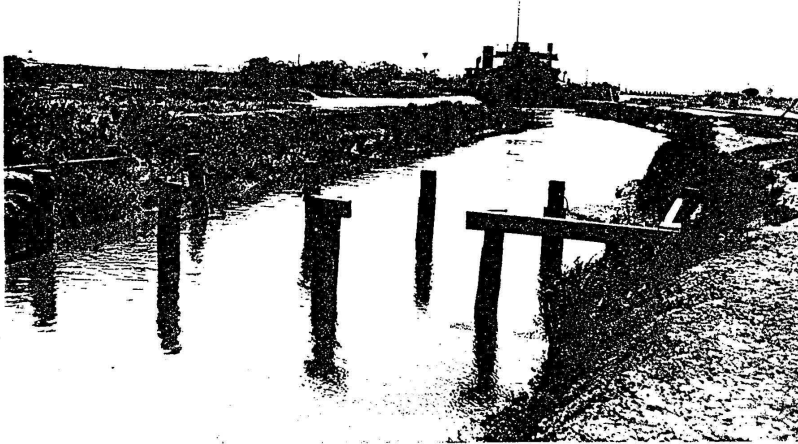
PLATE 4-7 The constructed outlet of Moonee Ponds Creek partially blocked by the dredge "Lady Stanley" 12 January 1934. The piles in the foreground are all that remains of one of the temporary bridges that were washed away during the Christmas Day flood of 1933
