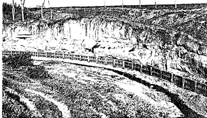
PLATE 4-12 Eroded bank and retaining fence built by the MMBW Reynard Street, Pascoe Vale 1934
