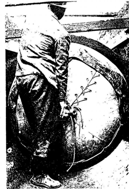
PLATE 4-17 The pneumatic core process. Locality unknown
