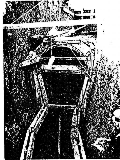
A Royal Park Drain: Outlet at Moonee Ponds Creek
