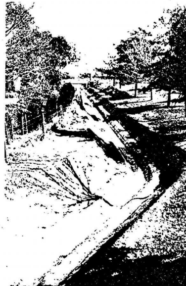
D Upstream from Napier Street after construction
