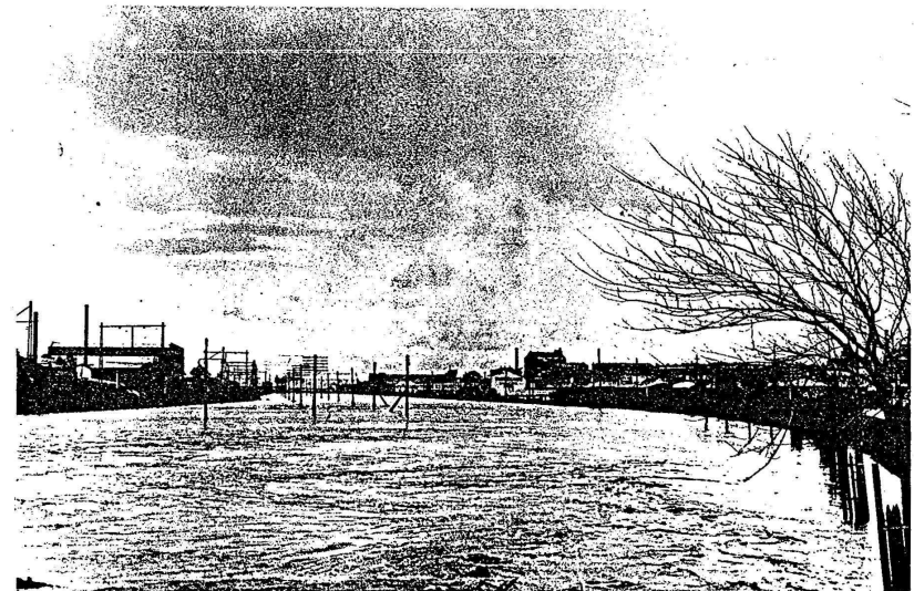
B View looking downstream from Racecourse Road Bridge
