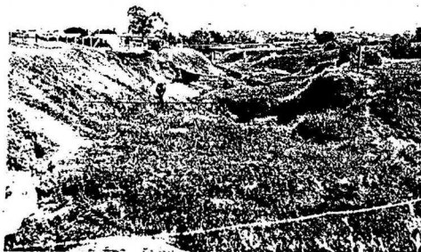
MELVILLE CREEK AT McLEAN STREET BRIDGE
