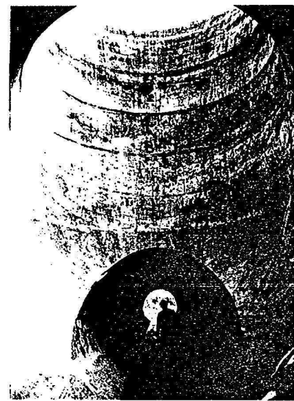
B The entry of the glory hole spillway into the normal outlet pipe
